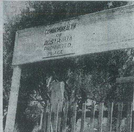
This fence has been repaired.
