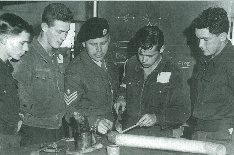
Apprentice Plumbers Balcombe 1956 - learning to solder downpipe
