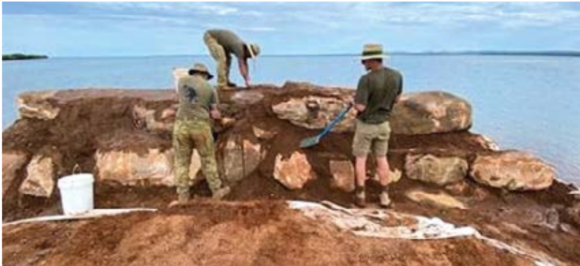
OP Resolute – ECN 411 and 412 technicians building a landing point for a barge to allow support
