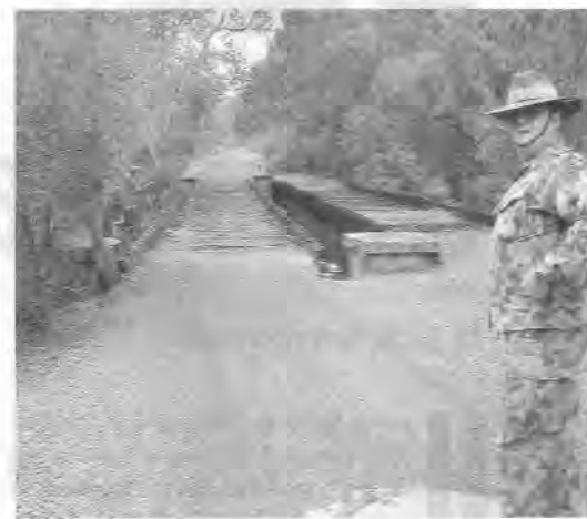
Old rail bridge
